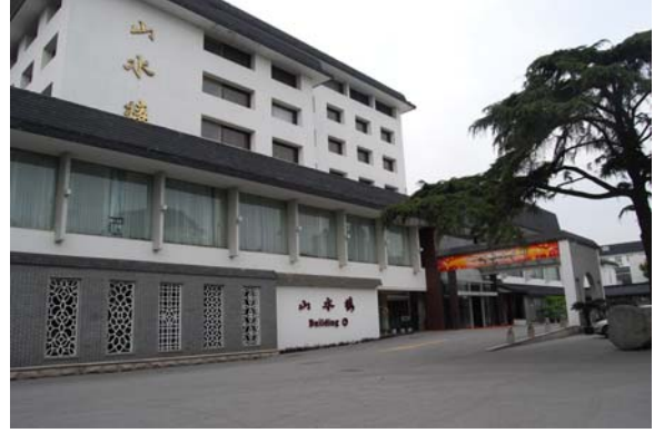
Building 2 of Nanlin Hotel (Shanshui)
